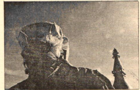
The veiled head of the Statue of Guru Padmasambhava under construction in Samye Monastery prior to its demolition by PAP. The photo was taken in January by unknown person. ©TCHRD
