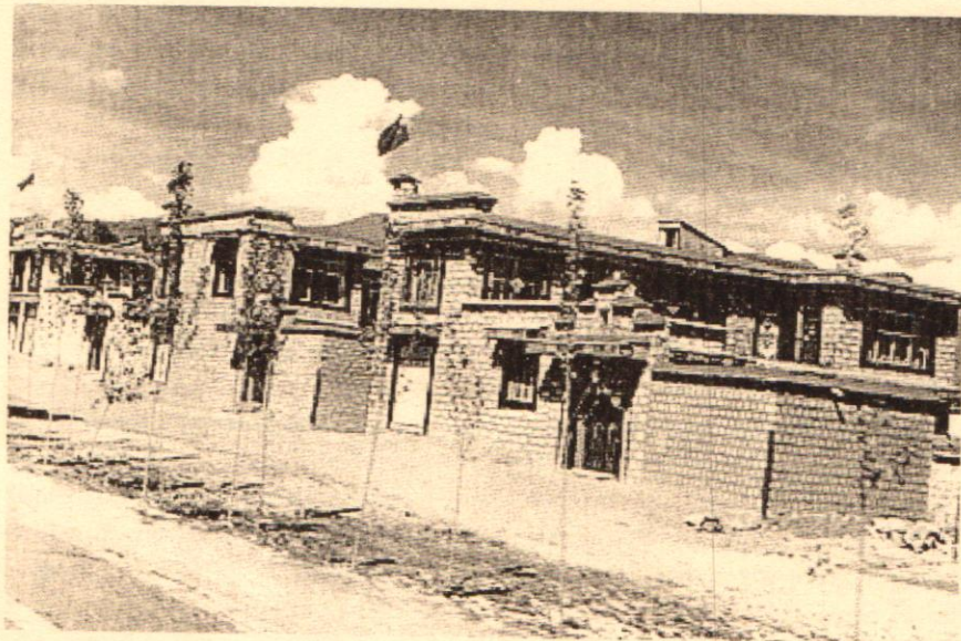
New House constructed in rural Tibet.
