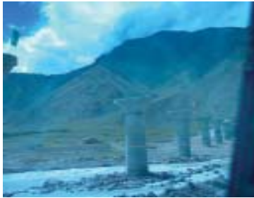
Bridge under construction over Toelung River near Lhasa © Tashi Wangdu
