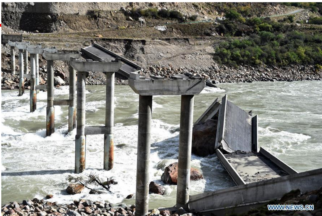
Dalin bridge, damaged by rushing water from a landslide-caused barrier lake on the Yarlung Tsangpo River in Menling County (Xinhua/Chogo)
